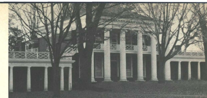
The massive two-story, six-column portico of Pavilion V at the university is generally considered the most impressive of the pavilion facades. It is Ionic, after Palladio. Like all of the Pavilions, it was originally designed with a study and "lecturing room" — as Jefferson called it — on the main floor, living quarters for the professor's family above and kitchen, laundry and storage space below. (Photo by the author.)
