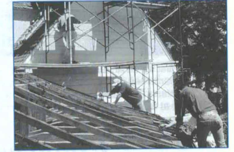
16 George Washington's Mansion has been undergoing renovation.
