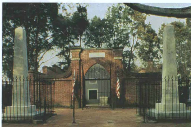
The "New Tomb" as ordered in Washington's will was not constructed until 1831. He had selected the site, but left no known design. Records indicate that Robert E. Lee, a young army engineer, was involved in the Tomb's construction. While George and Martha Washington rest peacefully in sarcophagi in the vestibule, 20 other members of the family are buried in the vault.
