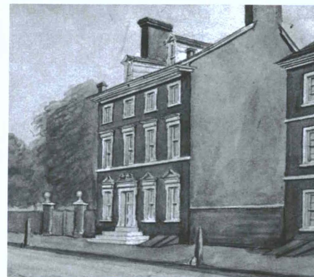
President and Mrs. Washington lived, during his term of office, in this residence owned by Robert Morris at 190 High Street in Philadelphia. President Adams also resided here until moving to Washington, DC in 1800. Original watercolor rendered by W. L. Breton. (Courtesy the Historical Society of Pennsylvania.)
