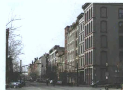
Main Street boasts an array of cast-iron storefronts just south of the river.
